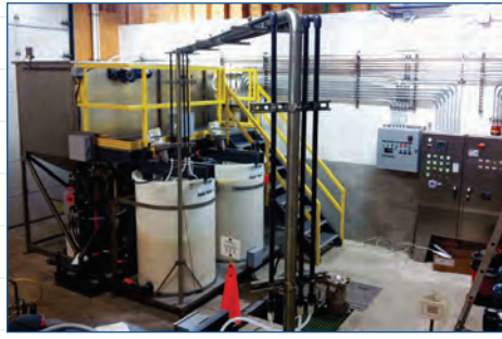
Continuous flotation wastewater treatment system (5 – 1,000 gal. per minute).
